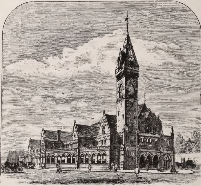
Boston and Providence Railroad Depot, Columbus Avenue.
